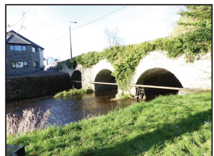
Image 010: Rathangan Bridge from south
