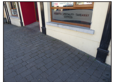
Image 006: Ramped surfaces on Bridge Street
