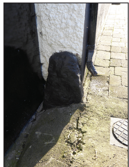
Image 024: Wheel fender and threshold
