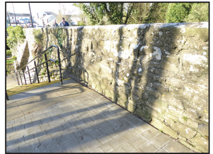
Image 018: Existing surfacing and parapet wall
