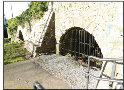
Image 021: Abutments and bridge arch
